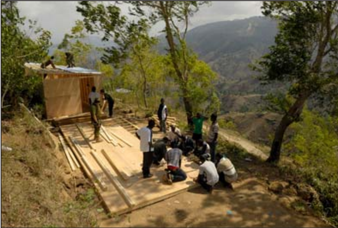
Disaster Assistance Response Team (DART) members and local workers assemble the floor of a shelter being constructed at an orphanage in Fondwa, Haiti. (Canadian Forces photo by Master Corporal David Hardwick)
